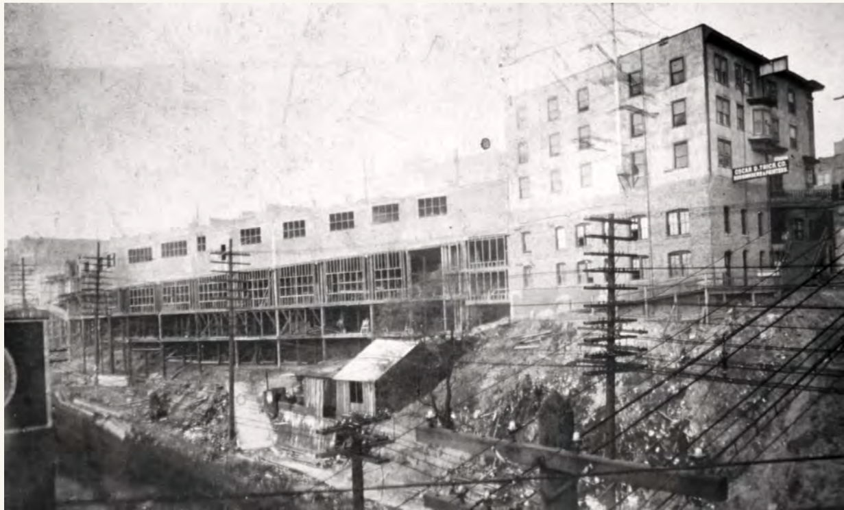
The construction of the lower levels around 1914. (Seattle Municipal Archives)
