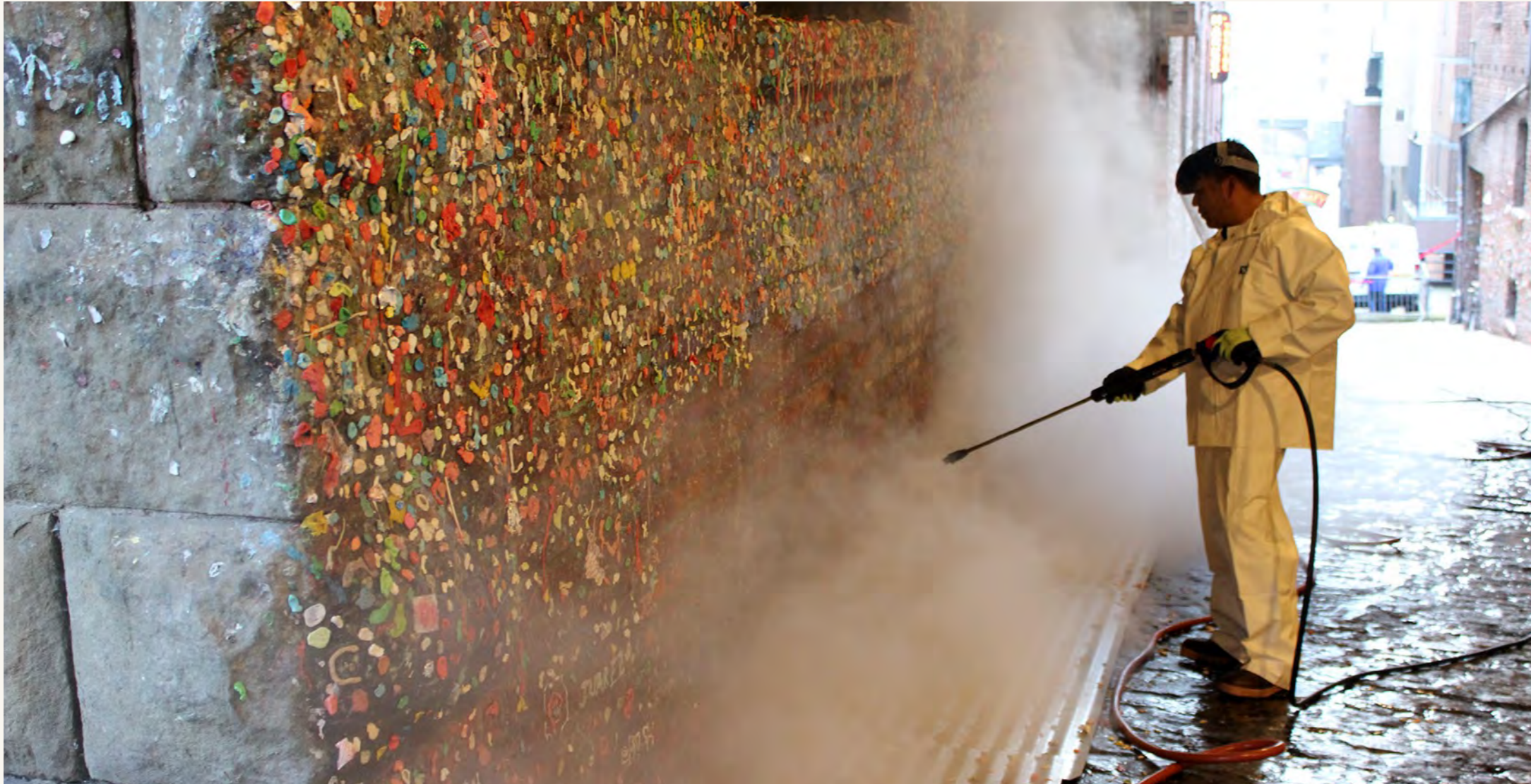
The PDA contracts annual cleaning of the walls in lower Post Alley, using pressurized steam. Quarterly maintenance prevents the Gum Wall from spreading beyond its origins next to the Market Theatre. (PDA)
