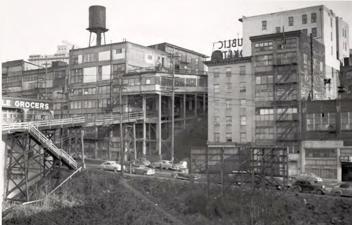
A view of the back of the Market from the Alaskan Way Viaduct in 1951. (Seattle Municipal Archives)
