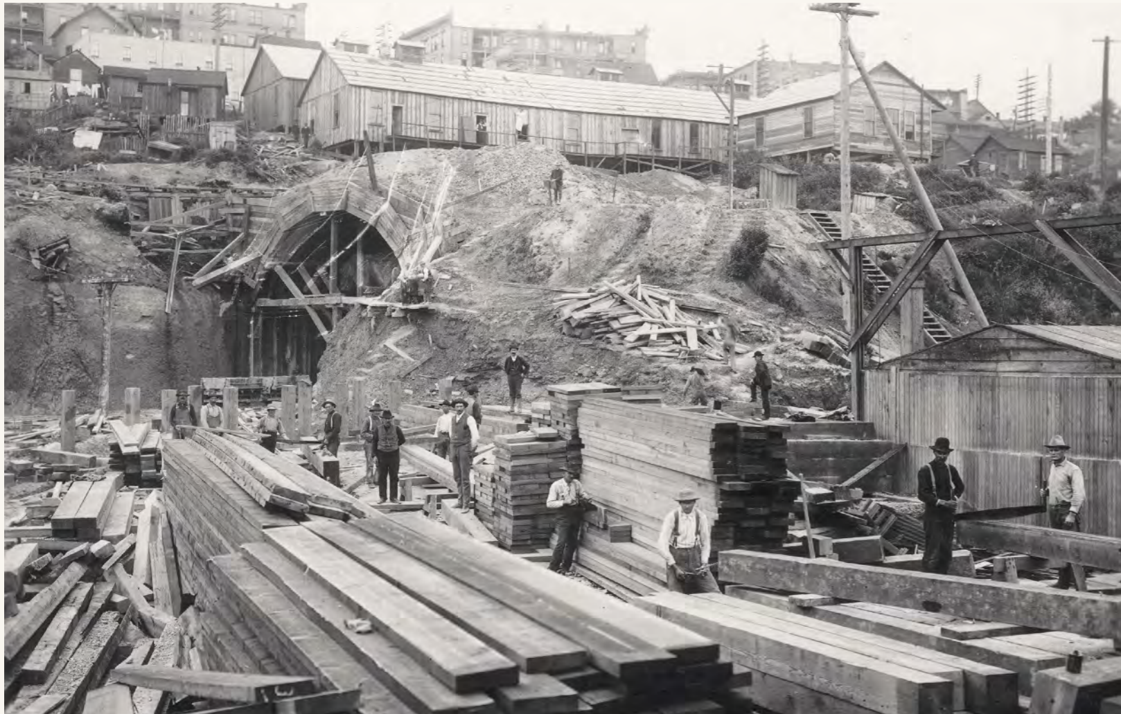
Workers' housing can be seen in the top of this 1903 photo, above the construction site of the tunnel, dug by hand between 1903 and 1905. (Asahel Curtis, University of Washington Special Collections)
