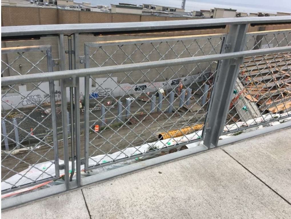
Typical screen railing at overlook.
