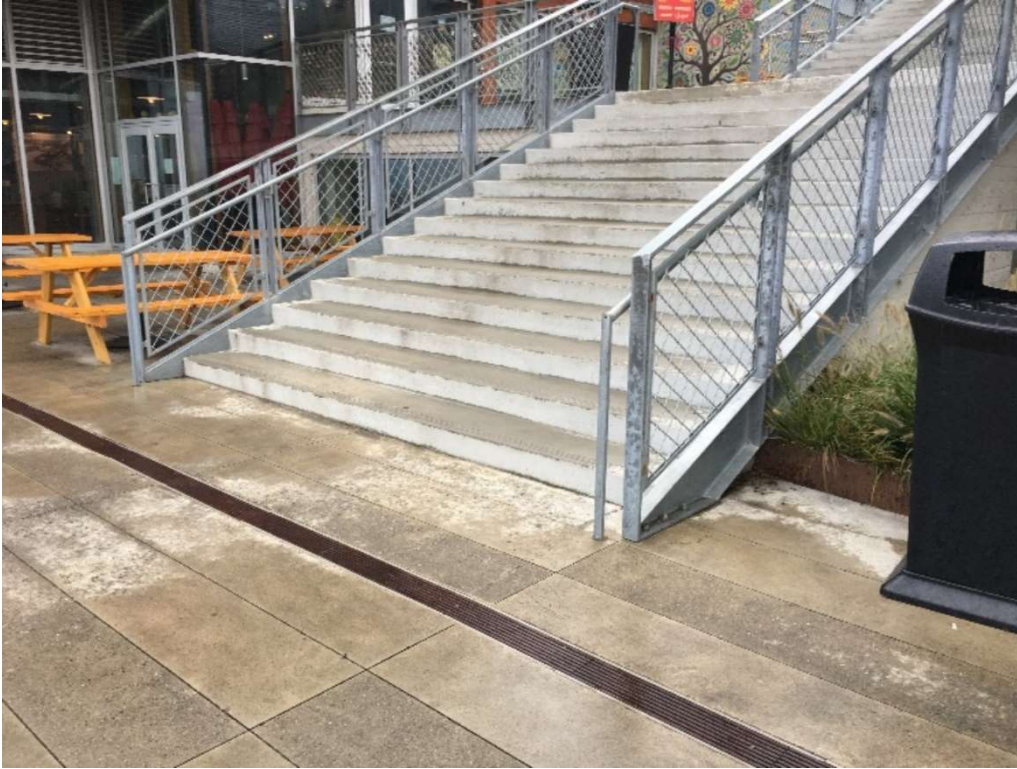
Screen railing at stair.
