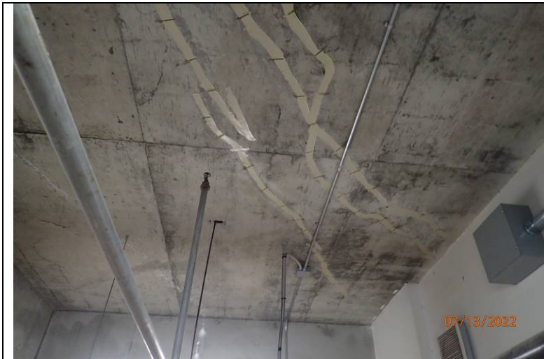
Photograph 22: Injection performed in the ceiling of the food bank.
