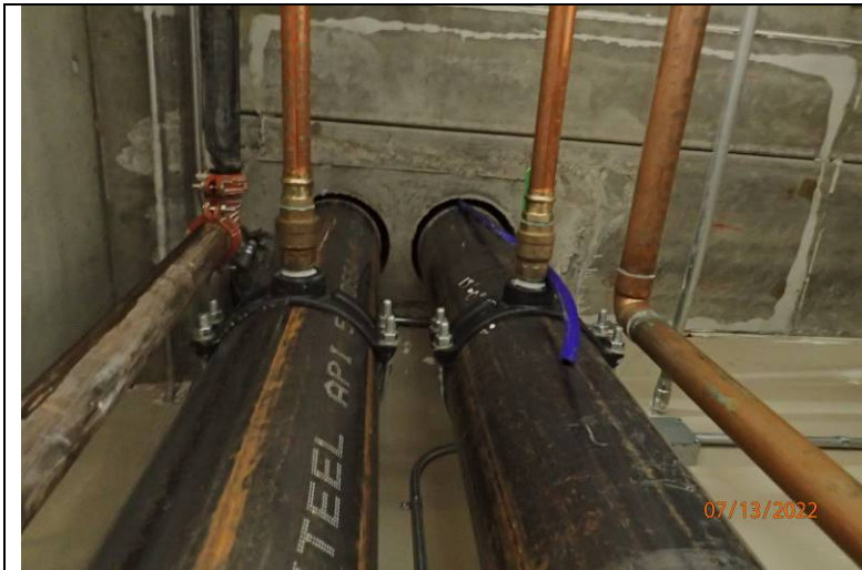
Photograph 25: Closer view of the chiller line penetrations through the concrete.
