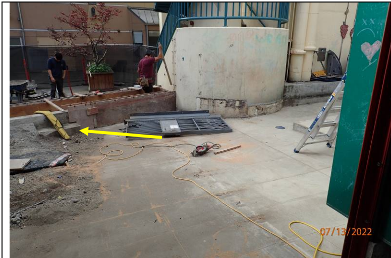
Photograph 19: Looking south at the north end of the plaza and area of work by SSI. The slope of the plaza is to the left (east) and through drainage mat that travels under the concrete stem wall. The drainage mat will be restored and installed under the new finishes over the topping slab visible in this photo. Arrow shows direction of water flow.
