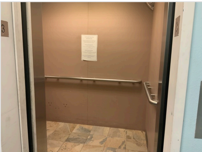
Lobby looking at cabs (with doors open)
