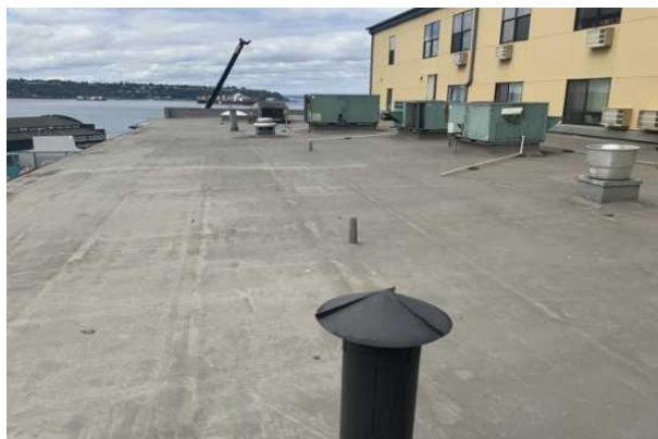
6 PRIMARY ROOF OVERVIEW
