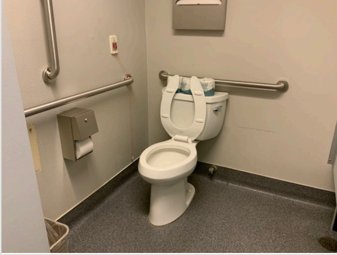
Toilet stall overview
